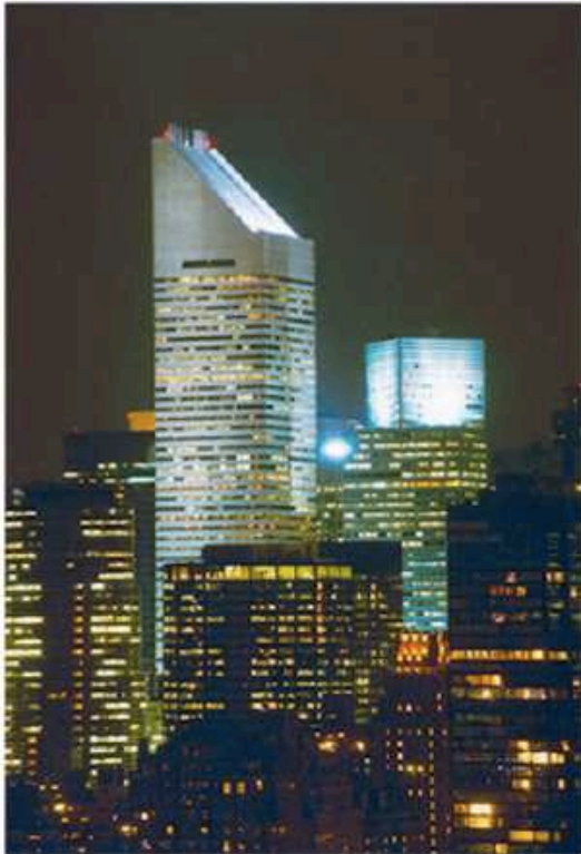
fig 5b. Citigroup Center, completed 1977 architect Hugh Stubbins Jr. 153 E. 53rd St., New York
